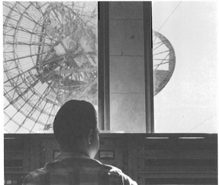
Operations room of Apollo-Goldstone tracking station was in direct contact with Apollo 8 during the most critical phases of the journey via the 85-foot antenna above. The station, a key site in NASA's worldwide network of Apollo facilities, houses approximately 160 six-foot racks of electronic gear.
